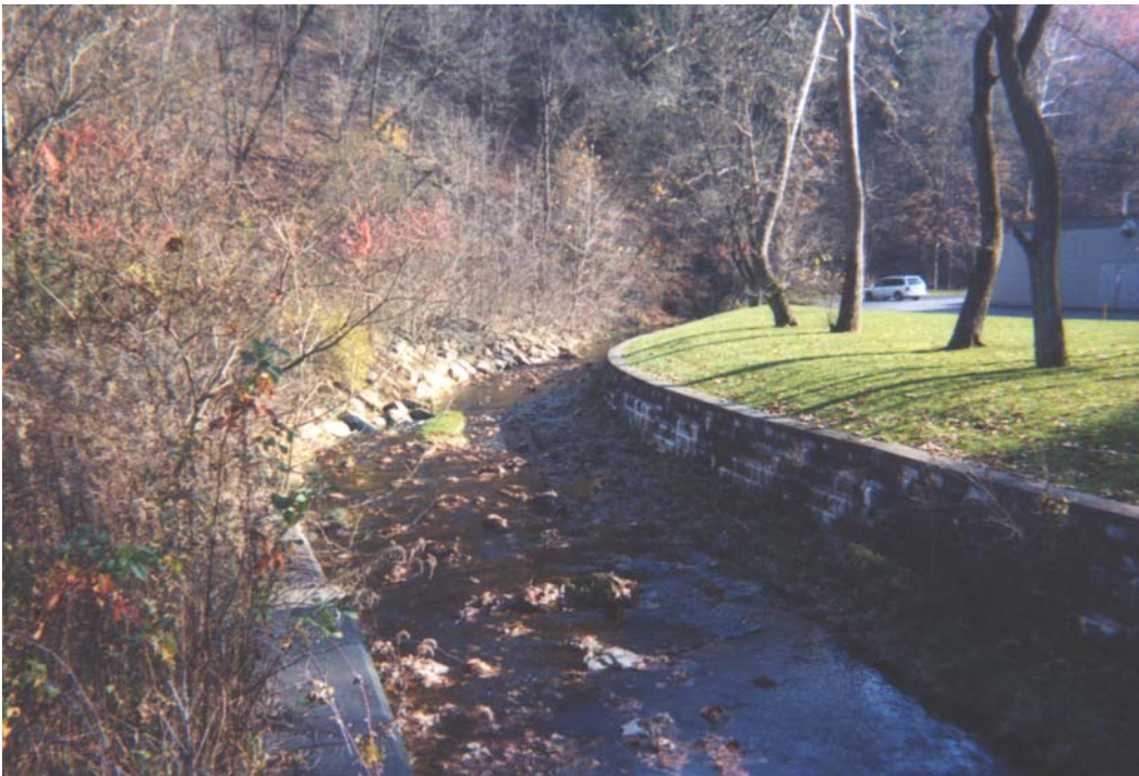
Figure 6.8: Photo of Little Pine Creek at watershed outlet
