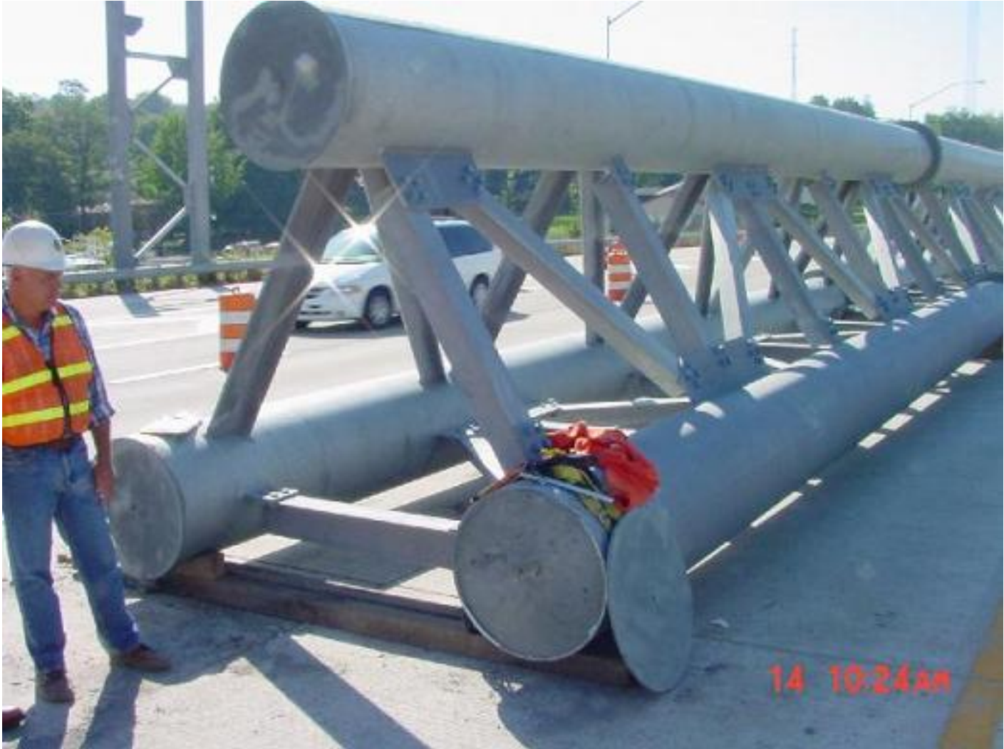
Figure 1 Tri-Chord Overhead Sign Structure
