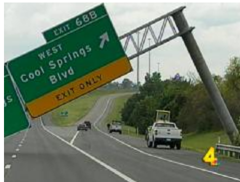
Figure 1-1 Collapse of cantilevered structure along I-65 in Tennessee
