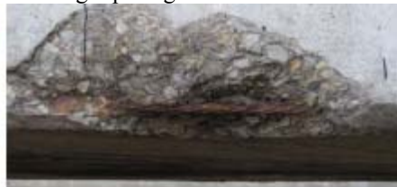
(e) corroded strand with heavy pitting.
