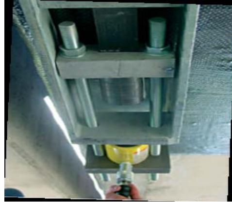
(b) jacking end anchor in movable frame.
