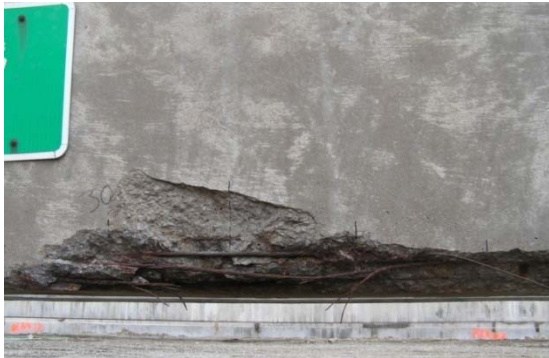
Figure 3-4 Exposed and ruptured strand due to vehicle impact (Lake View Drive Bridge; Harries 2006).
