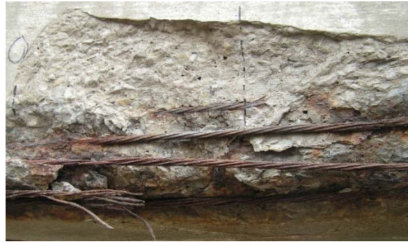
Figure 3-4 Exposed and ruptured strand due to vehicle impact (Lake View Drive Bridge; Harries 2006).
