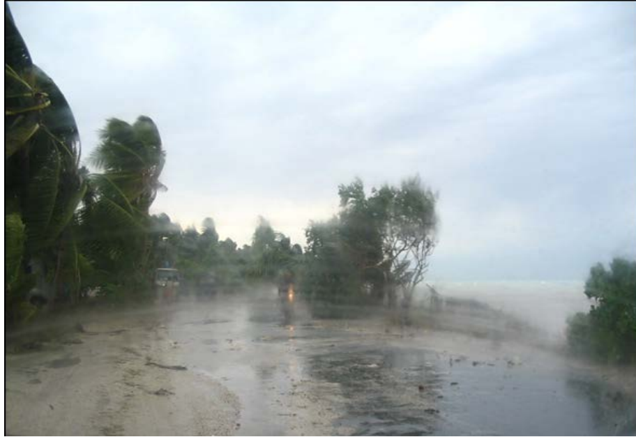
Figure 15. King Tides Washing Over a Road, Tarawa, Kiribati
