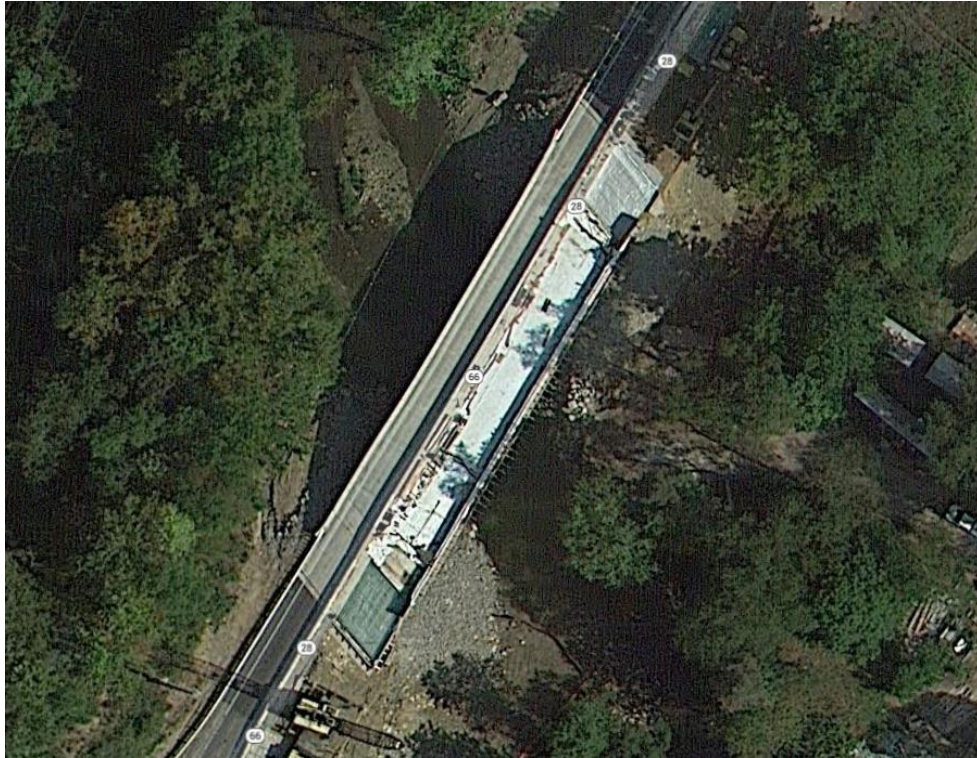
Figure C118: Bridge on SR0028 over Cowanshannock Creek
