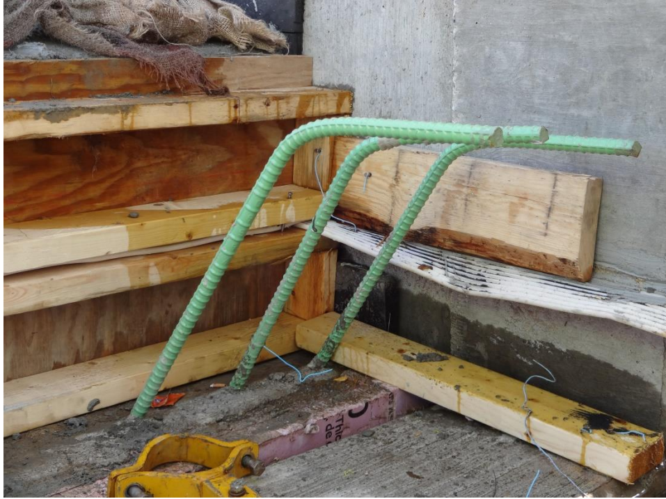
Figure C116: Waterstop extended to curb overlapping on additional piece of waterstop
