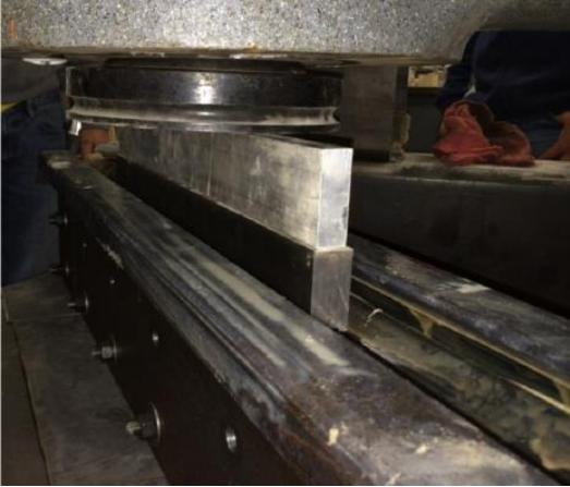
Figure 3.12: Loading of strip seal
