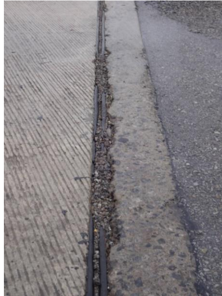
Figure 4.17: Clear visibility of compression seal joint – Prospect #1 Bridge
