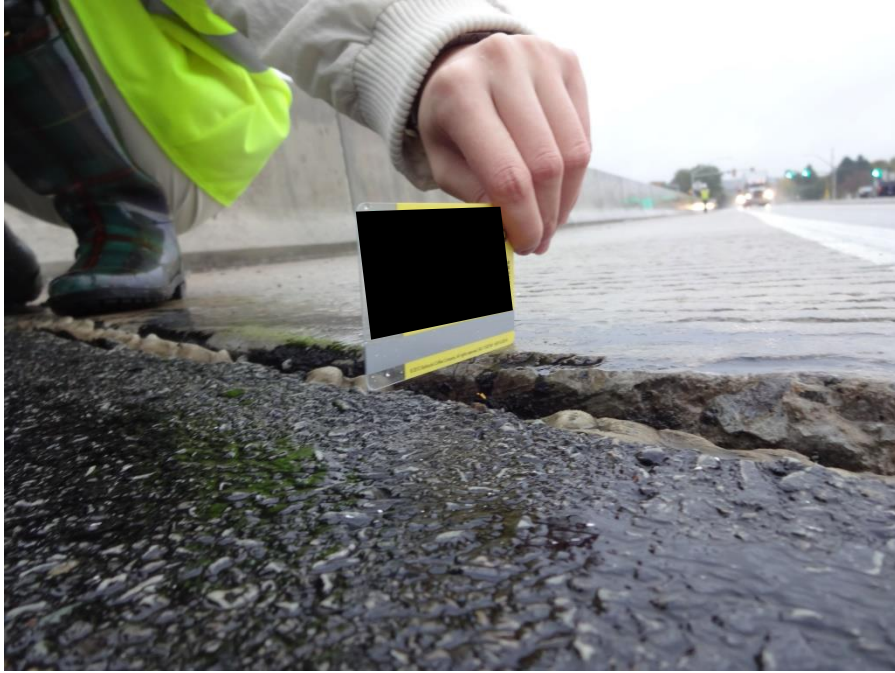
Figure C71: Interface of bridge deck and approach slab
