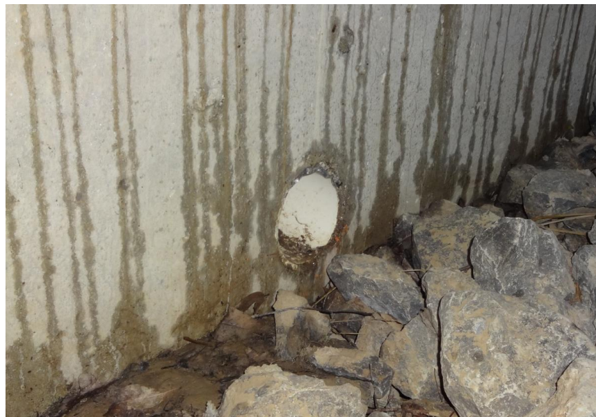
Figure C104: Weep hole on retaining wall
