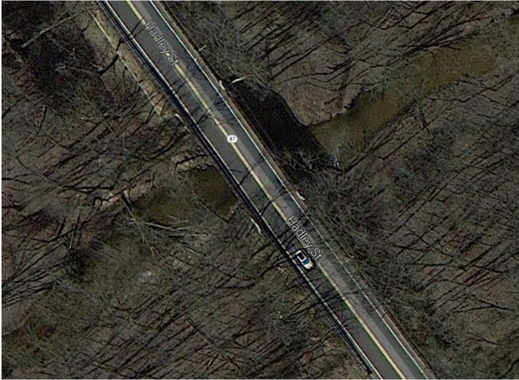
Figure C122: South Hadley Bridge
