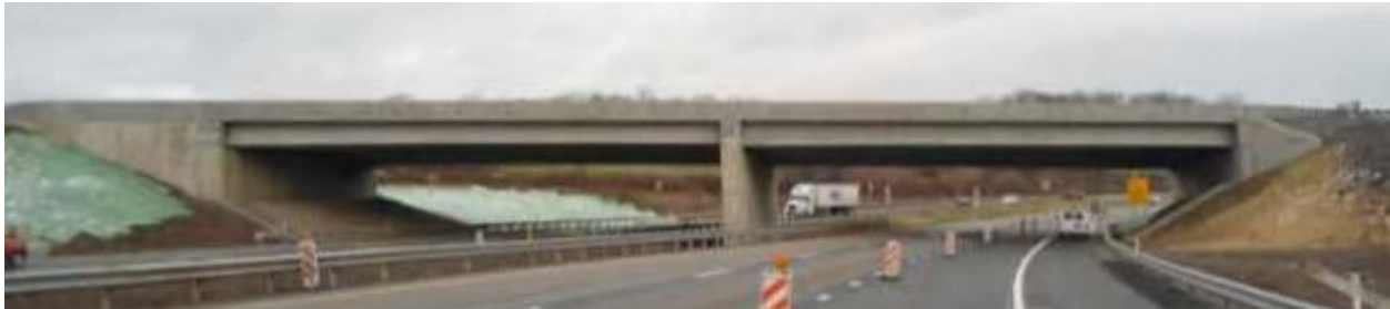
Figure 3.1: Little Creek Road Bridge
