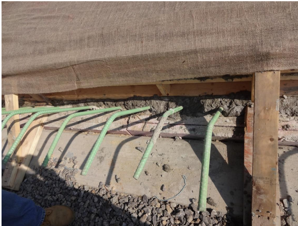
Figure C117: Polystyrene foam fillers in between approach slab and bridge deck
