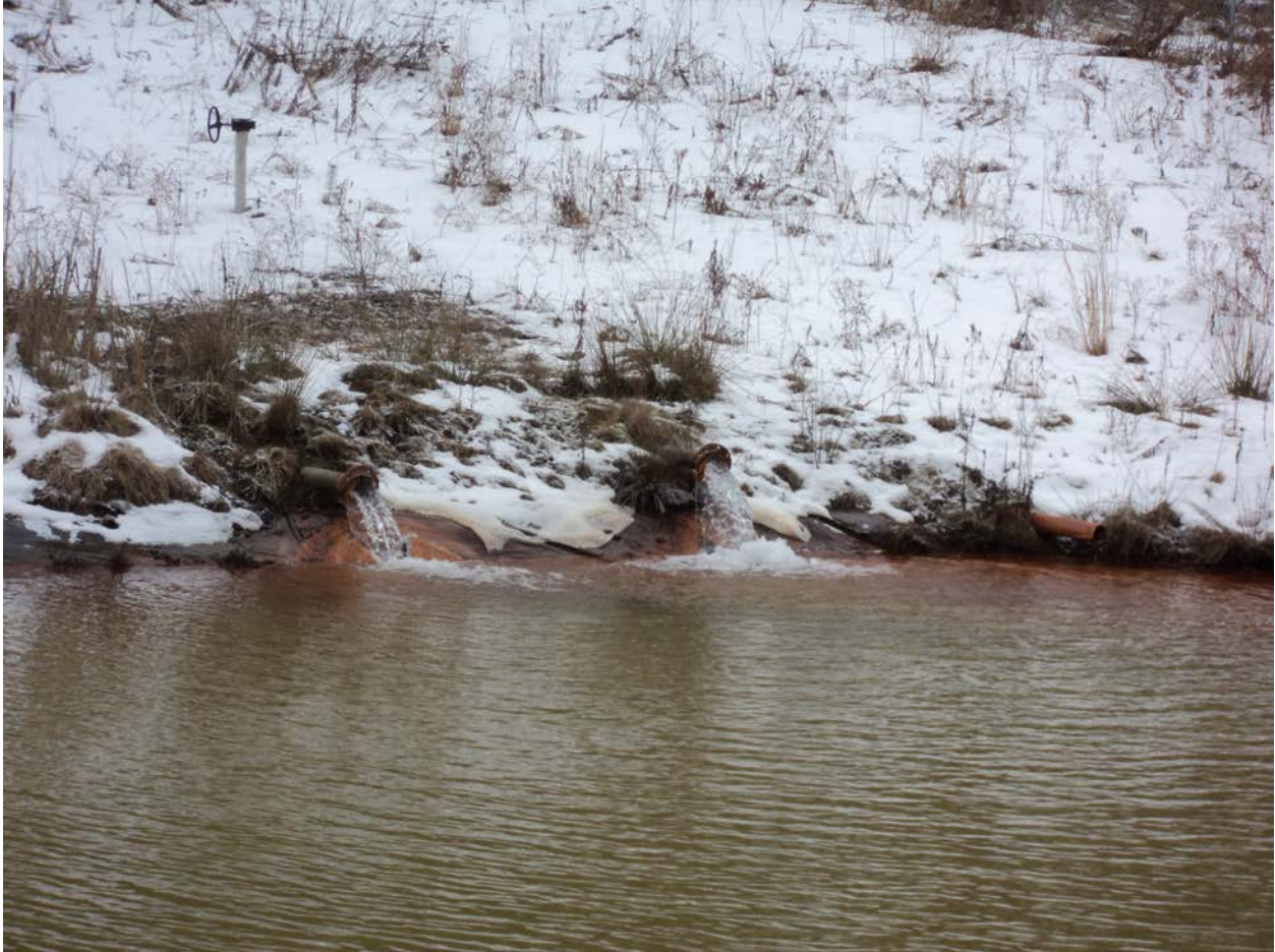
Figure 4.14 Horizontal borehole inflow to the Dora 6 settling pond near Perrysville Run.
