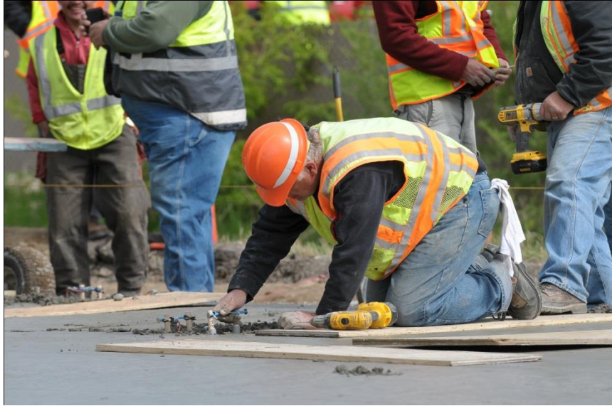
Figure 3.6: Installing Upper Layer Sensors after Passage of First Paver
