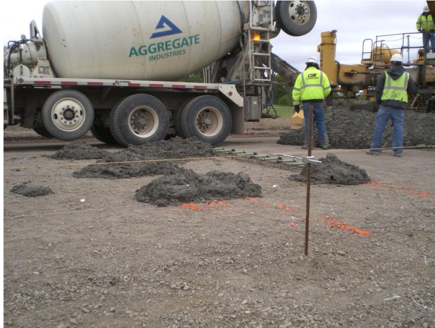
Figure 3.5: Paving Operations and Concrete Covered Sensors - Cell 70
