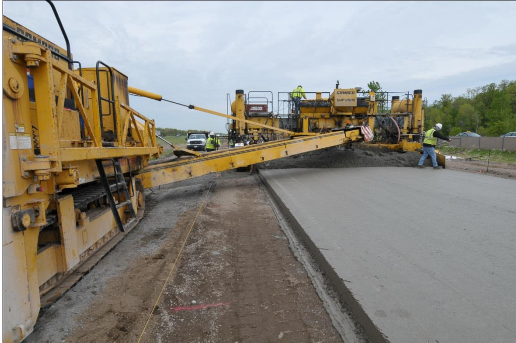
Figure 3.7: Placement of Upper EAC Lift
