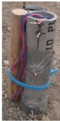
Figure 3.10: Thermocouples Installed at MnROAD
