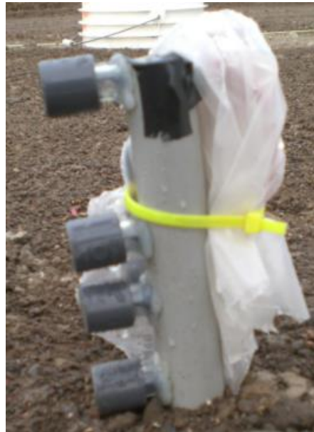
Figure 3.14: Relative Humidity Sensor Installation at MnROAD
