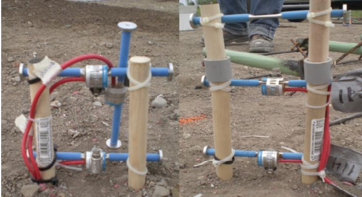
Figure 3.16: Vibrating Wire Installation - Cells 71 and 72
