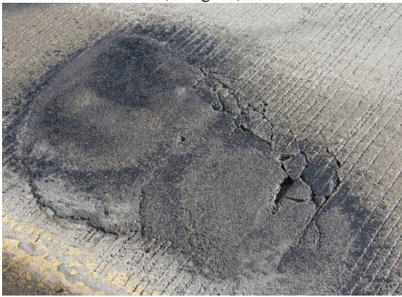
c) Mortar Patch of LMC (Bridge F)
