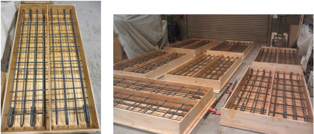
Figure 10: Laboratory Slab Forms Prior to Placing Concrete
