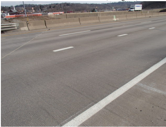
c) LMC Overlaid Deck of Bridge C (photo taken 1.14.13)
