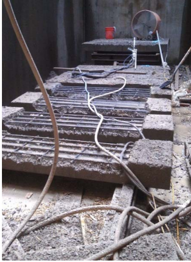
a) Slabs During Hydrodemolition
