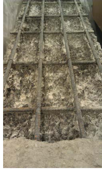
b.) Hydrodemolished Surface Profile
