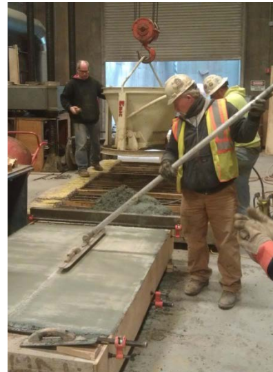
d) Installing LMC Overlay
