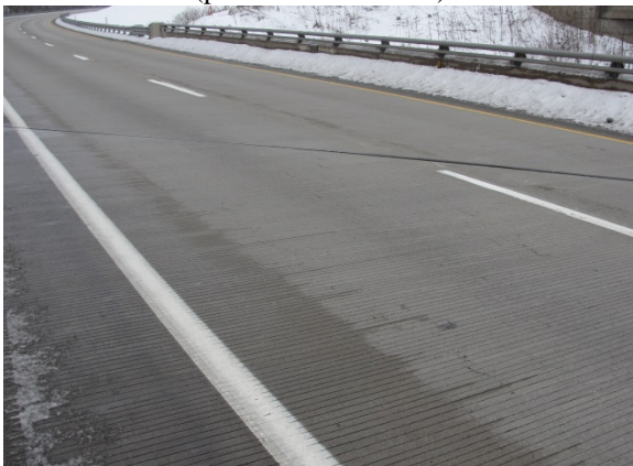
e) LMC Overlaid Deck of Bridge E
