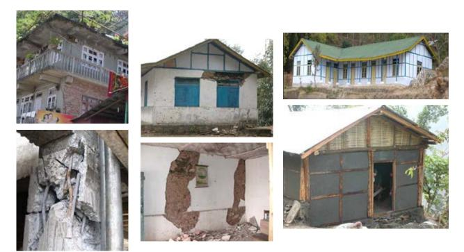
a) damaged concrete structure b) damaged masonry structure c) traditional Ikra structure **Figure 2-16: Typical** residential structures following the 2006 Sikkim earthquake (Kaushik et al. 2006)
