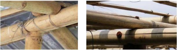
(a) Beam splitting at joint (b) Splitting at bolted connections Figure 4-1: Examples of bamboo splitting (Sharma 2010)
