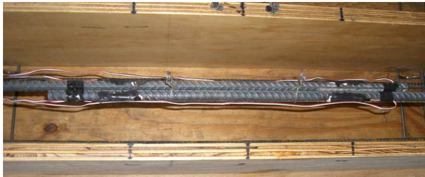
(e) Photograph of lap splice for Beam C-S-18.
