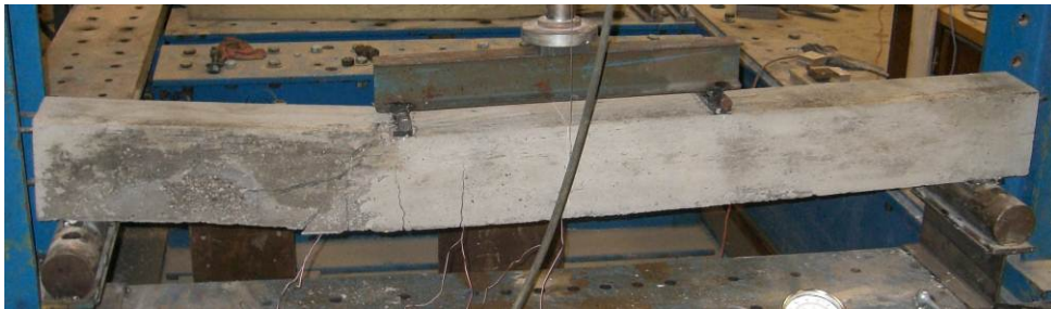
Figure 2.17 Photograph of beam S-18 cracking after failure.
