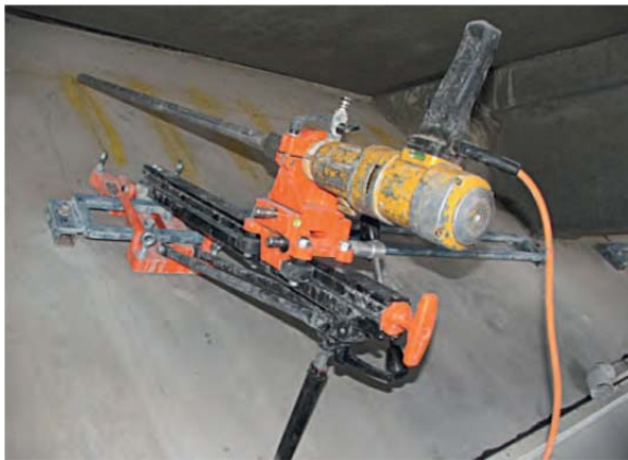
(a) Drilling chase in inclined concrete web.
