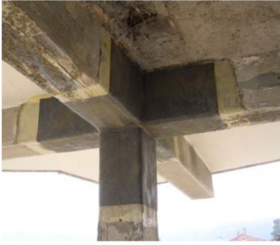
(a) Shear reinforced beam-column joint.
