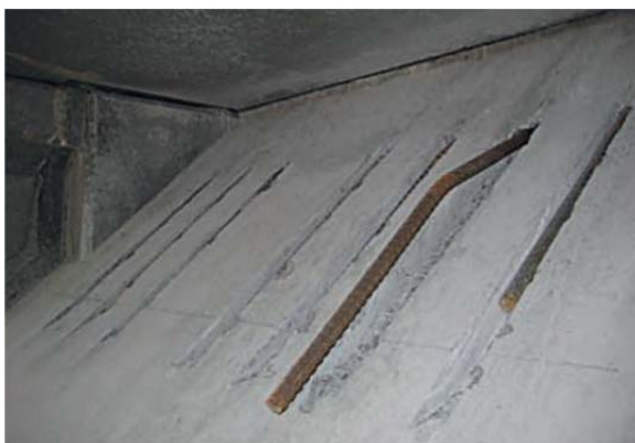
(c) 20 mm bar installed in chase.
