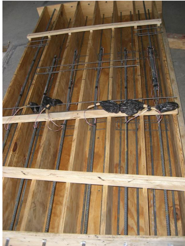
Figure 2.1 Arrangement of forms prior to casting concrete.
