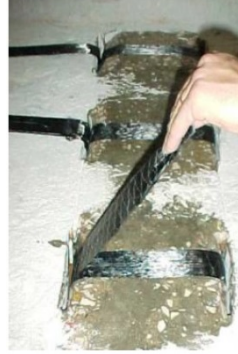
(b) Wrapping CFRP strips through slab.
