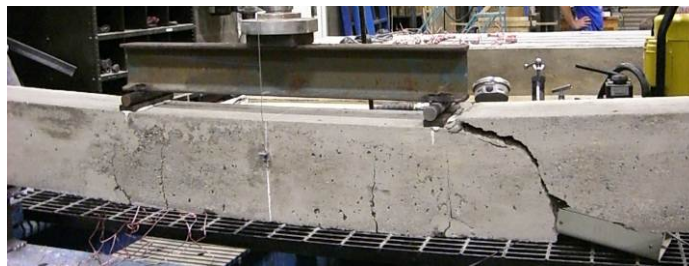
Figure 2.14 Photograph of beam C-S-18 cracking after failure.
