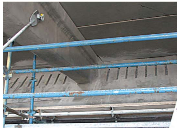
(b) Completed chases.
