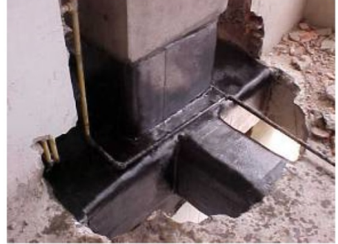
(c) Removal of concrete volume.
