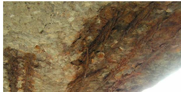
d) Typical corrosion of strands resulting in significant loss of section at soffit of box girder.
