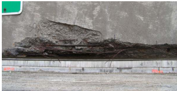
c) Typical damage to strand resulting from recent vehicle impact.
